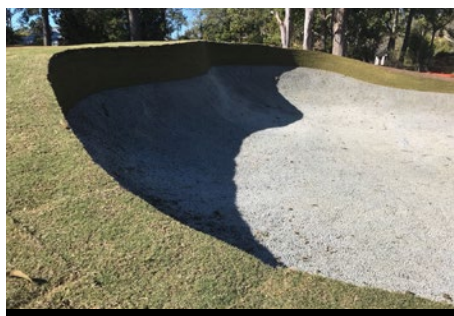
EcoBunker edges at Killara, Sydney. The sand belt style is now viable anywhere!
