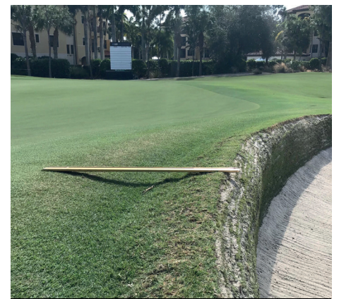
Hurricane Damaged Bunker walls are being systematically removed.
